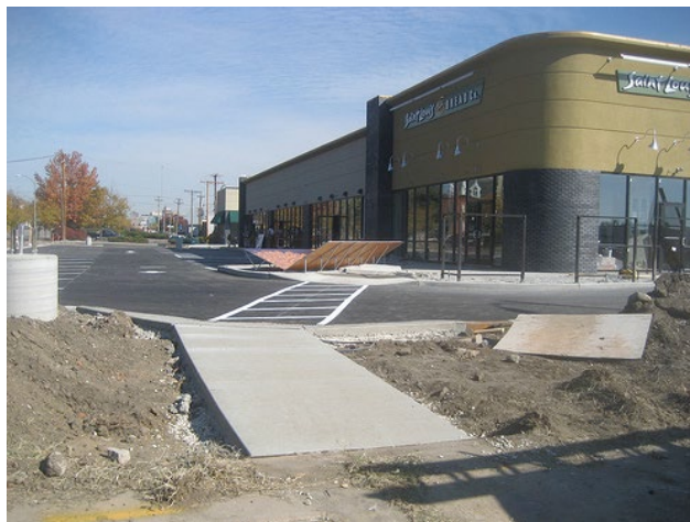
Figure 3.303-1: This image illustrates a sidewalk connection between a building and a public sidewalk in the right-of-way. This connection includes both a separate sidewalk (foreground) and a connection delineated through a painted line (background).
